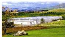
The Lindcove Protected Foundation Block (general view)
