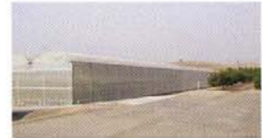
Protected Foundation Block
